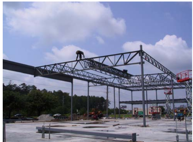
Figure 15 Shortspan joists being spread out along Joist Girder top chord by two Erectors
