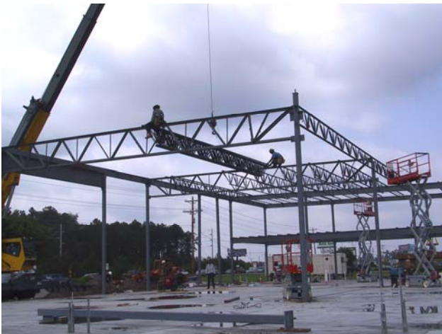
Figure 14 Bundle of shortspan joists being placed at mid-span of Joist Girders
