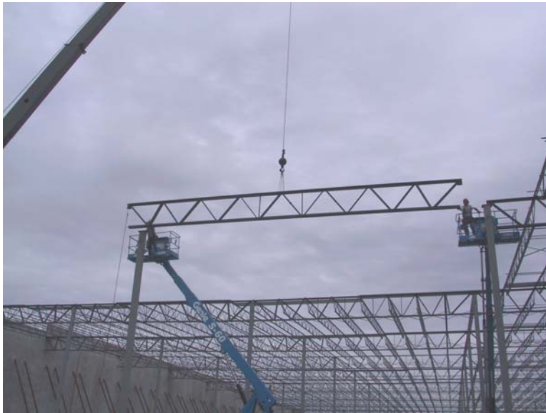
Figure 10 Joist Girder being set on two columns with two Connectors
