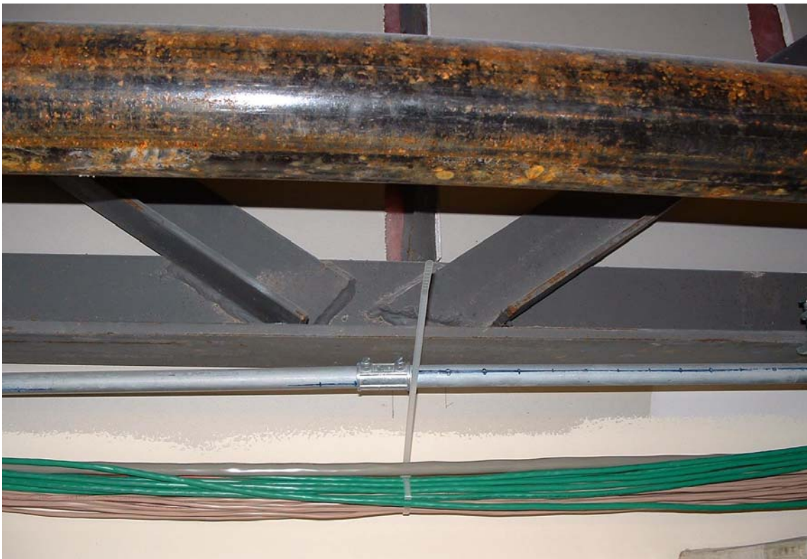
Fig. 14 Web Angles on Side of Chords
