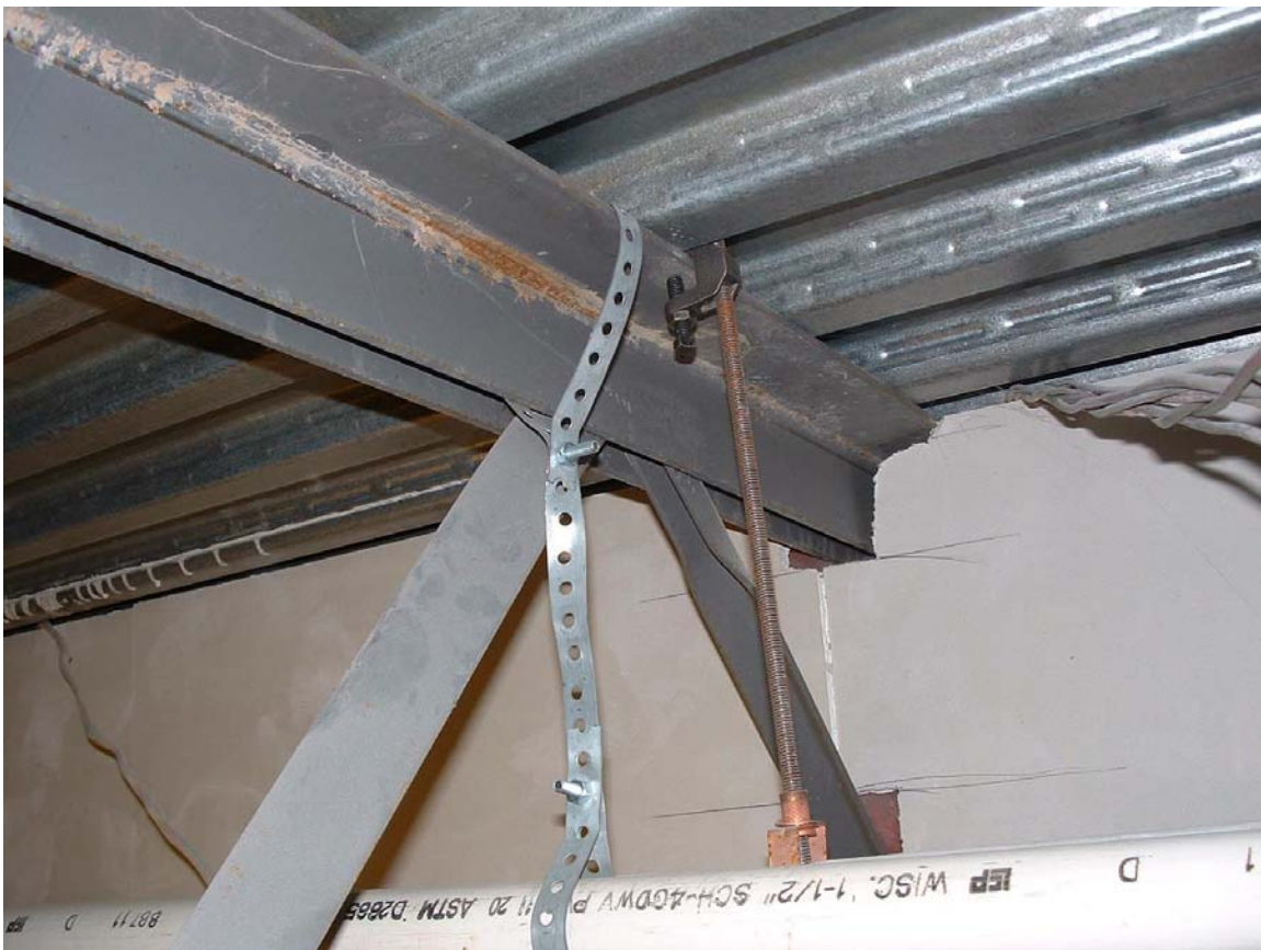
Fig. 7 Joist with Crimped Web Members.
