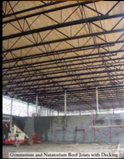
Gymnasium and Natatorium Roof Joists with Decking
