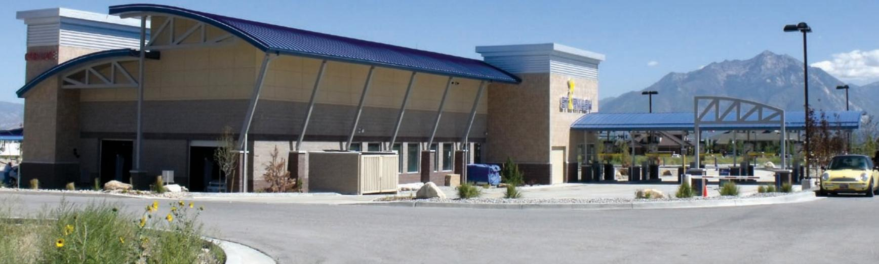
The Wasatch Range, which serves as a backdrop to the eco-friendly Star Wash car wash in South Jordan, Utah, inspired the facility's organic shape with multiple roof arches and open-web bowstring trusses and steel joists.
