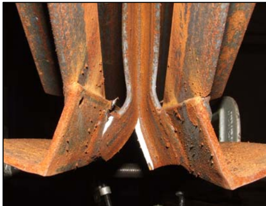
Figure 7 Weld and member fracture at the chord connection (J1175-W1)
