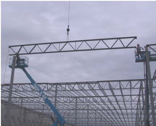
FIGURE 5 JOIST GIRDER BEING SET ON TWO COLUMNS WITH TWO CONNECTORS
