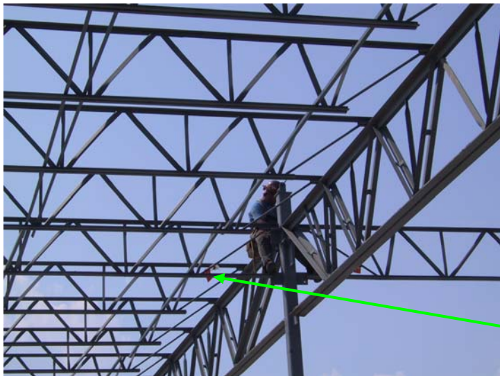
FIGURE 3 COLUMN JOIST BEING CONNECTED; BOTTOM CHORD IS “KNIFED IN” BETWEEN VERTICAL STABILIZER PLATE
